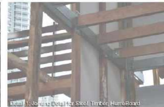
Detail 1: Jointing Detail for Steel, Timber, HumeBoard
