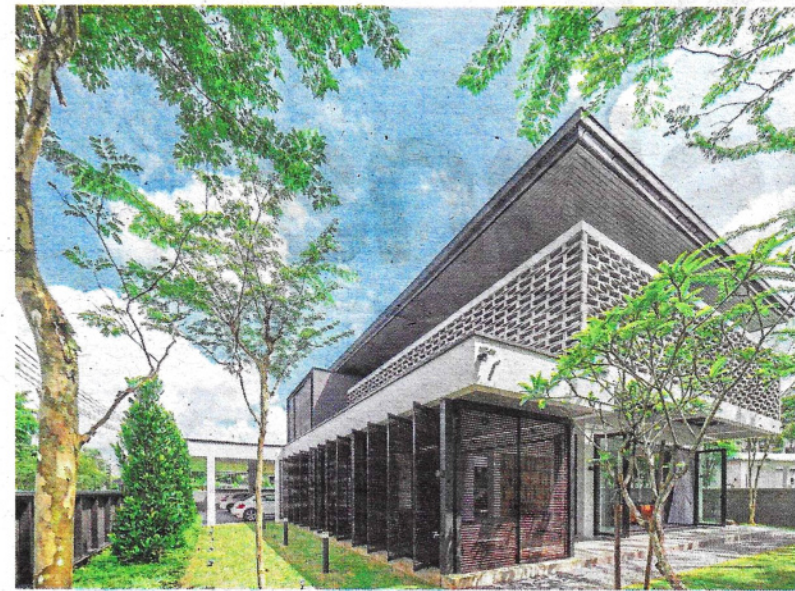
The vent blocks of the House at Urat Mata are meticulously arranged as a privacy screen that covers almost the entire first-floor exterior to strategically shade the upper dwelling from both the eastern and western sun. — MNSC Architects
