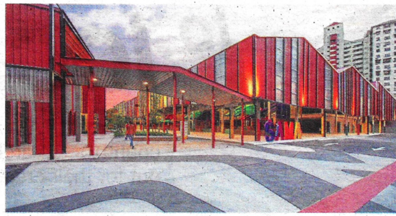
The drop-off area of SAMA Square's People's Plaza, which connects the sheltered tropical community market, food stalls and clustered landscaped retail space. — Tan Kwon Chong Architect
