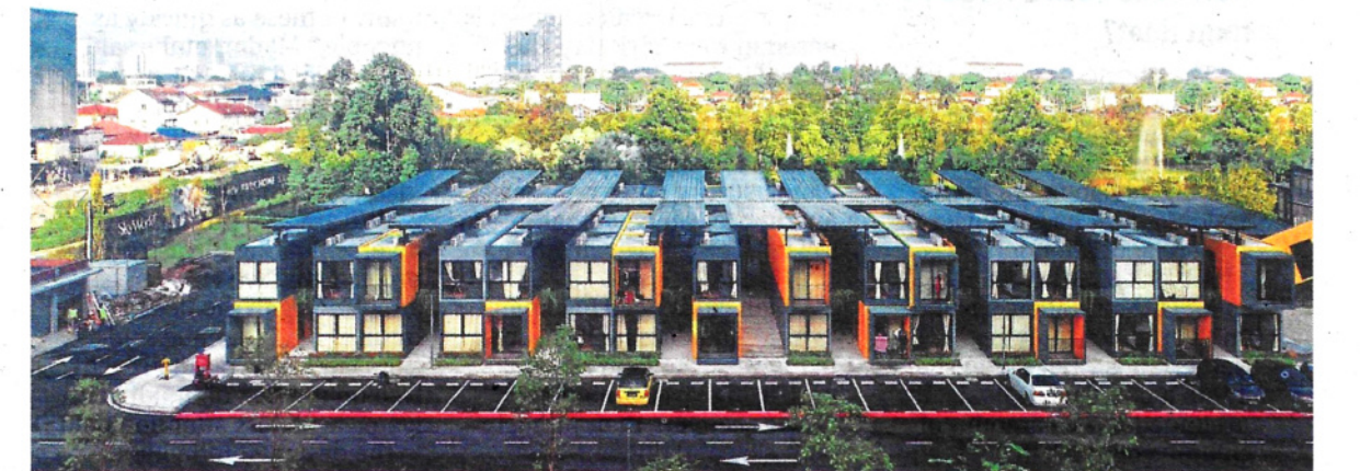
An overview of the vibrant yellow cantilevered Skyblox Co-Living Housing. — Pixelaw Photography
