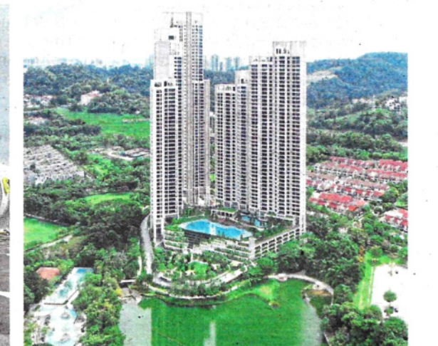
Park Regent, an example of urban integration, blends seamlessly with its landscape. — Environmental Design Practice
